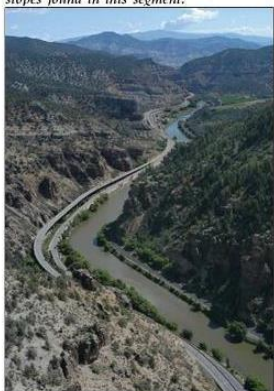
D | The roadway should respect the sinuosity of the valley floor and creek.
