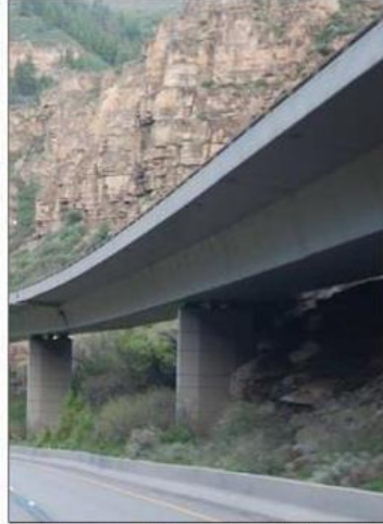
B | Deep overhangs and shadow lines add visual depth and give the bridge superstructure a thin appearance.
