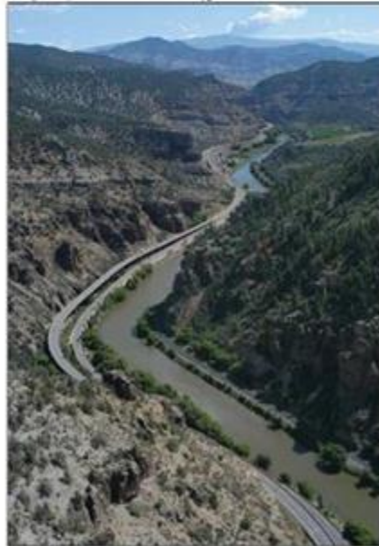
D | The roadway should respect the sinuosity of the valley floor and creek.
